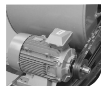
❶ Adjustable motor support bracket
