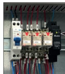
Leak detector power supply
