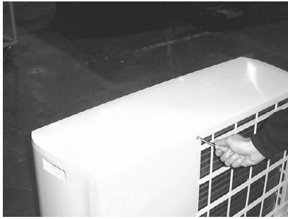
remove the middle screw (rear section)
